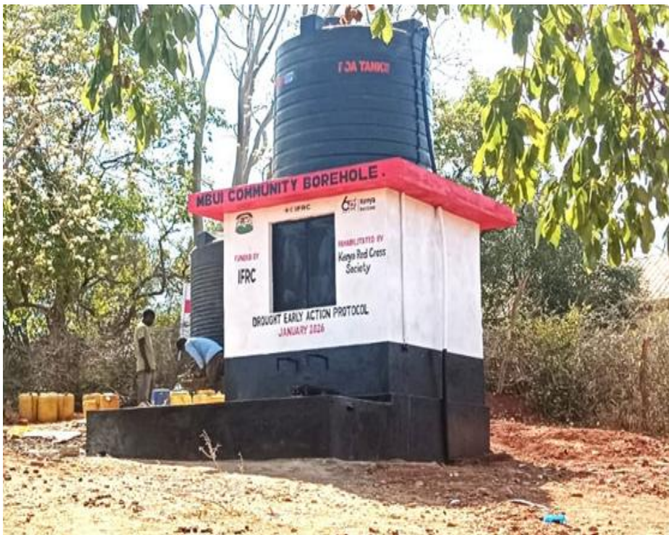
Rehabilitation and Pipeline Extension of Mbui Community Borehole in Kitui County
